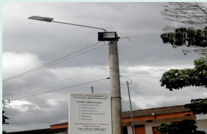
Newly installed street lights on a previously dark street
