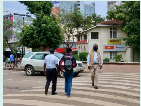
A wide raised pedestrian crossing that comfortably accommodates a large number of pedestrians, in Kisumu, Kenya
