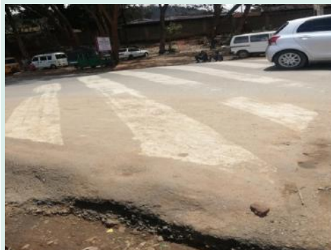
Newly erected and marked speed bump on the road along Machakos Primary school.
