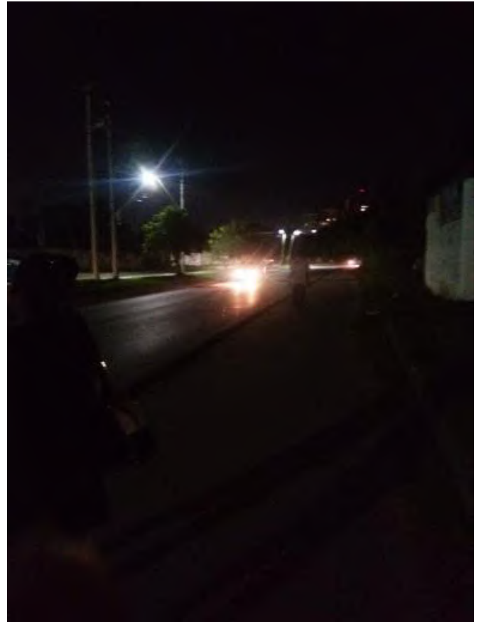
Image 2 showing one working streetlight on a road
